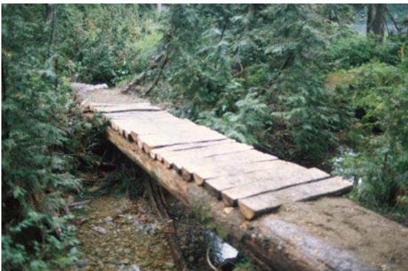
Y: Irregular surface trail with bog crossings
