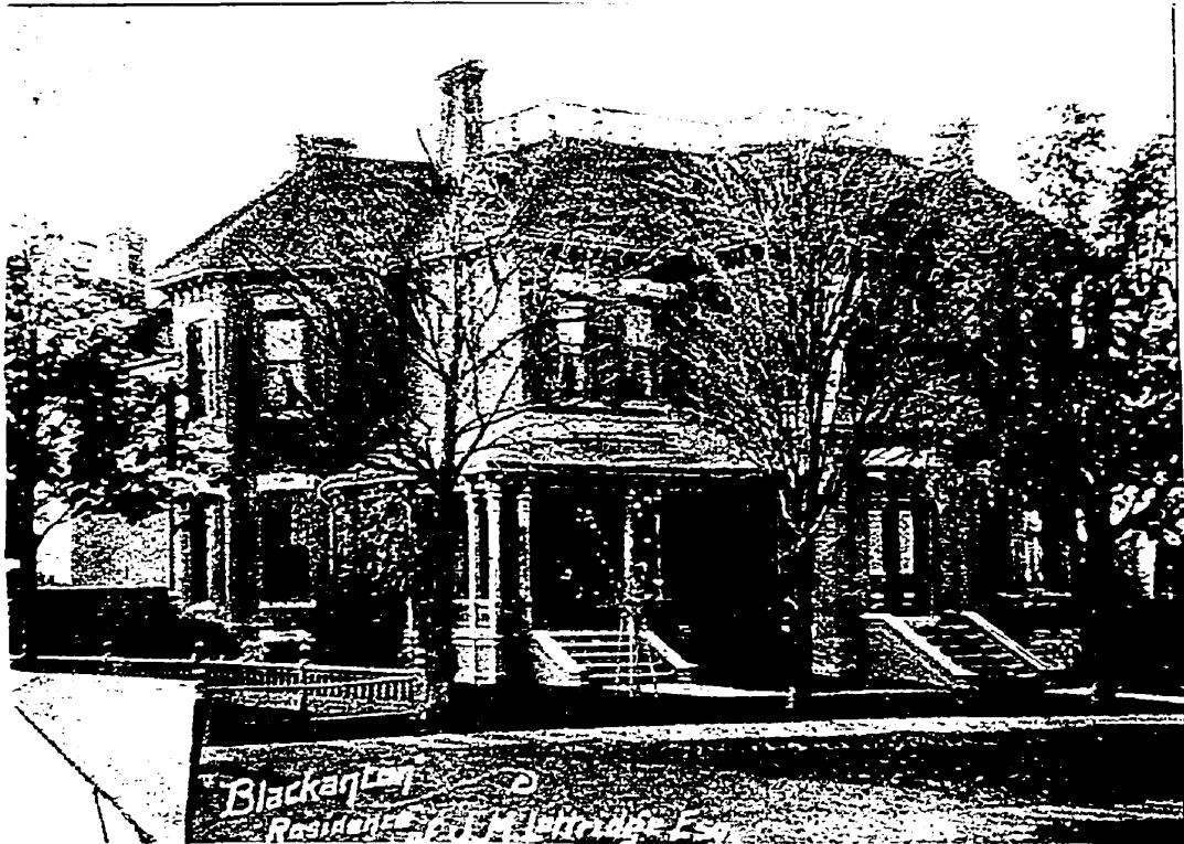
FIGURE 66: 301 Bay Street FIGURE 67: "Blackanton"
