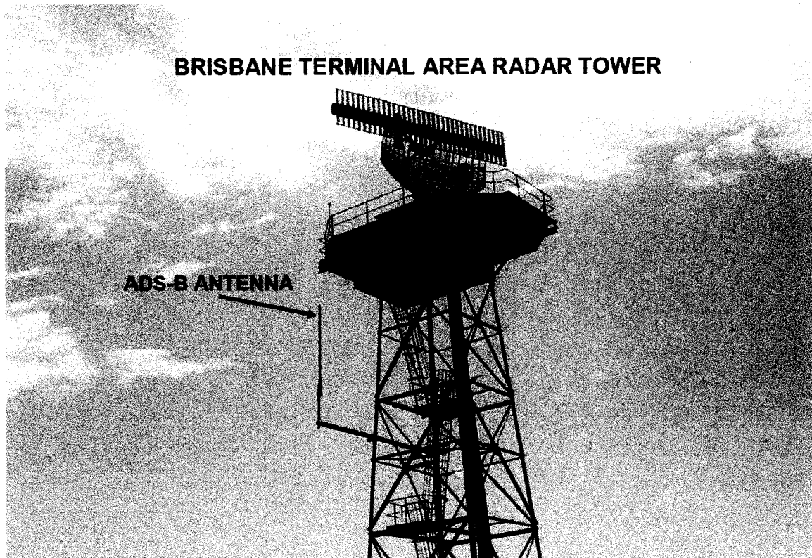
Figure 1.1: Comparison of ADS-B and radar antenna installations. Image from Dunstone (2005).
