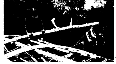
Bending inside chord of roundwood truss.
