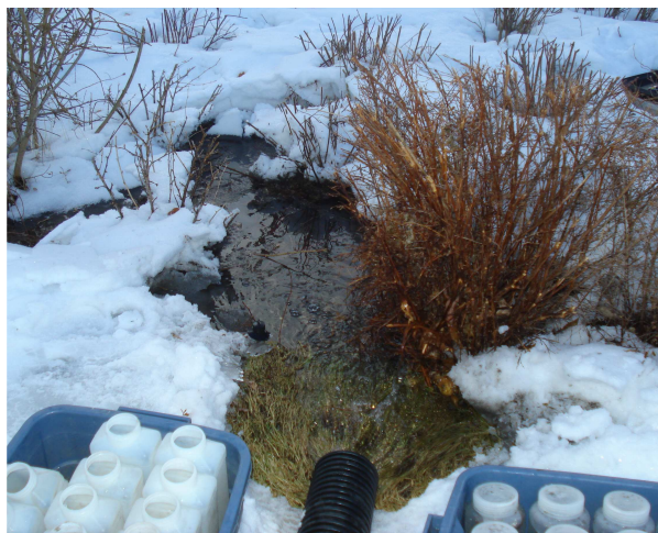
Figure 18: View of inlet of the bioretention cell in cold weather conditions
