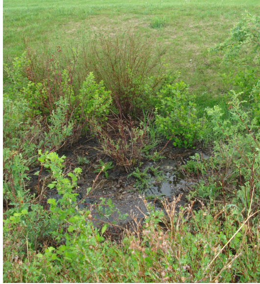
Figure 20: Ponding on the surface of the bioretention cell after an event
