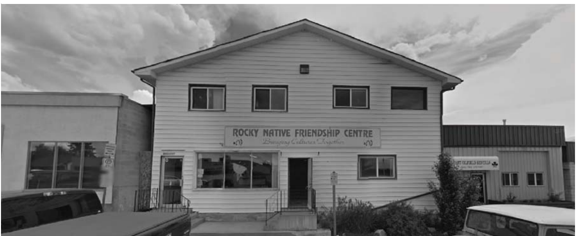
The Rocky Mountain House Friendship Centre, an example of adaptive re-use of a residential home. Rocky Mountain House, AB 2016; photograph from Alberta Friendship Centre Association website.
