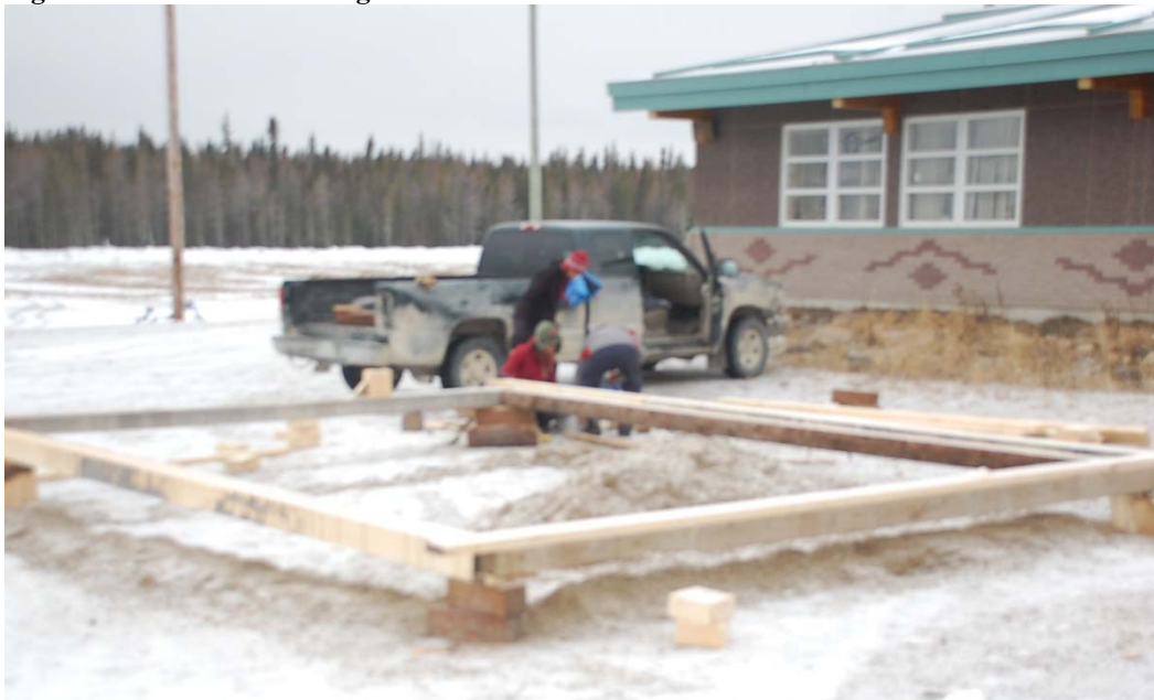
Figure 7.3: Foundation being built
