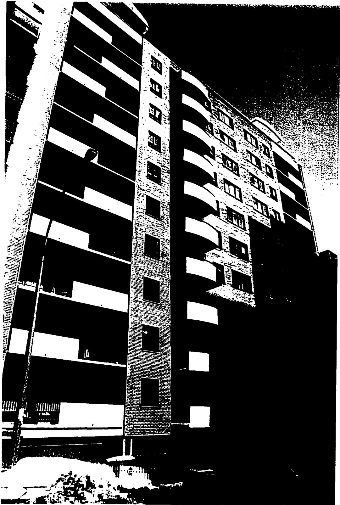
Fig. 14. Main Façade. Drummond Plaza Apartments, Montreal, 1957-8.
