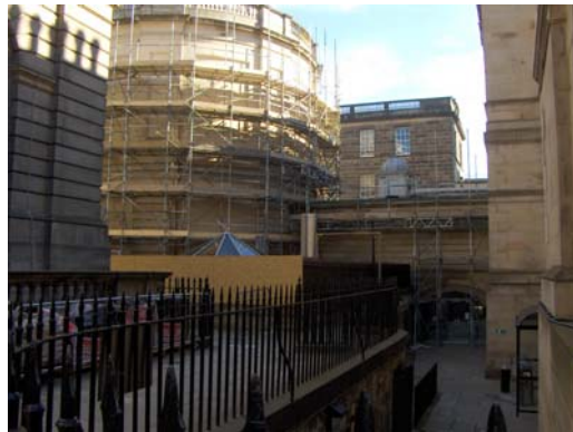
Figure 5.4: Scottish Family History Centre Under Construction, 2005
