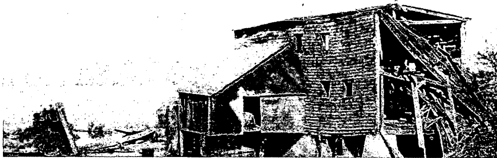
Ruins of Ramsay / Marchbank / Livingstone / Currie / Betts Sawmill on Little Pierre Jacques River, Glenwood, PEI, ca 1990. Photo courtesy Click Stewart.
