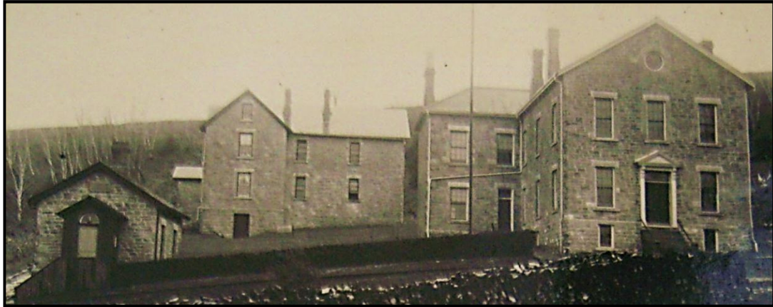
Figure 44: The Gore Bay Registry Office, Jail, and Courthouse, 1907 125
