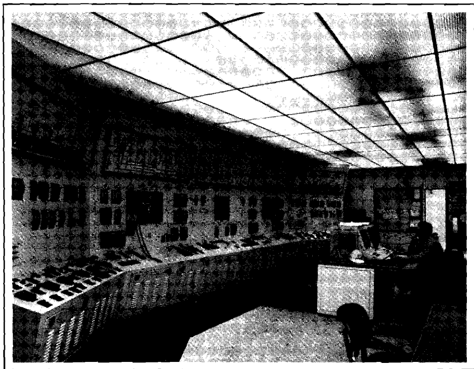
Figure 11. The central control room at the new Falconbridge Smelter, 1988. The intense use of technology in today's mining industry enables the operator in this room to monitor and control almost every stage of the smelting process. (Courtesy Falconbridge Ltd.)
