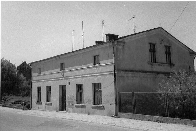
Photo 4.3. Soldau house with castle in background.
