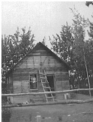
Photo 5.1. Dams' homestead farmhouse with ladder to attic.
